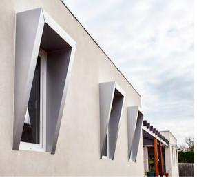
The owners have preferenced low-maintenance materials, such as aluminium-clad window shades (dubbed 'the eyebrows') over timber. They also chose screw piles instead of stumps to avoid use of concrete.
